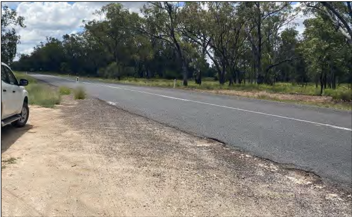
Figure 4: Kogan Condamine Road towards the west viewed from the intersection
